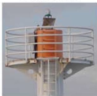
SL125-4 pylon installation, Israel
